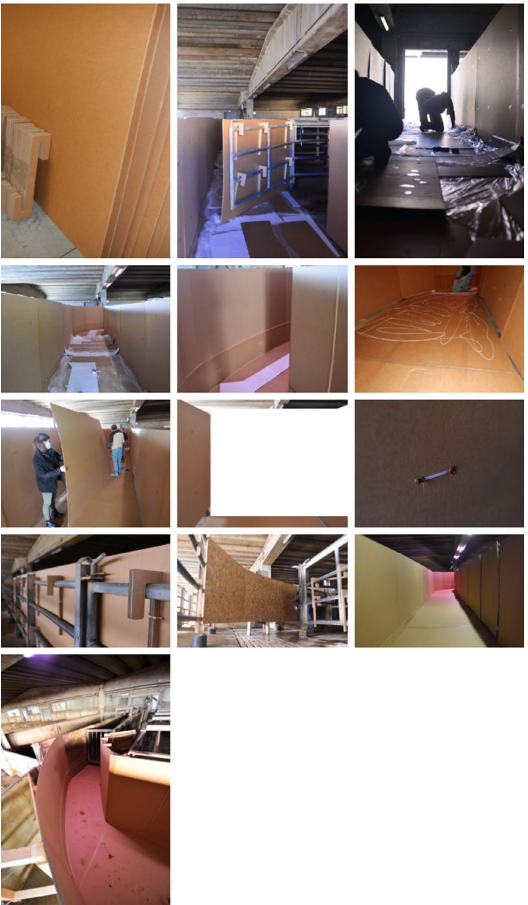
**PHOTOGRAPH 15** Photos showing the construction of the prototype. The utmost care was taken to ensure uniformity of the structure and to limit light infiltration through the use of adhesives of the same colour as the panels.
