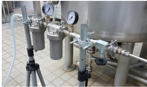
Stainless steel cartridge filters, 5 and 50 µm
